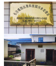
Integrated waste water treatment facility
