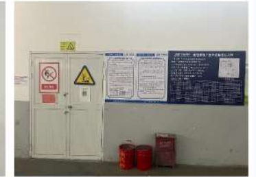
▲ Hazardous Waste Room
